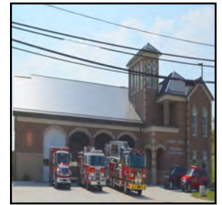
Central Fire Station
